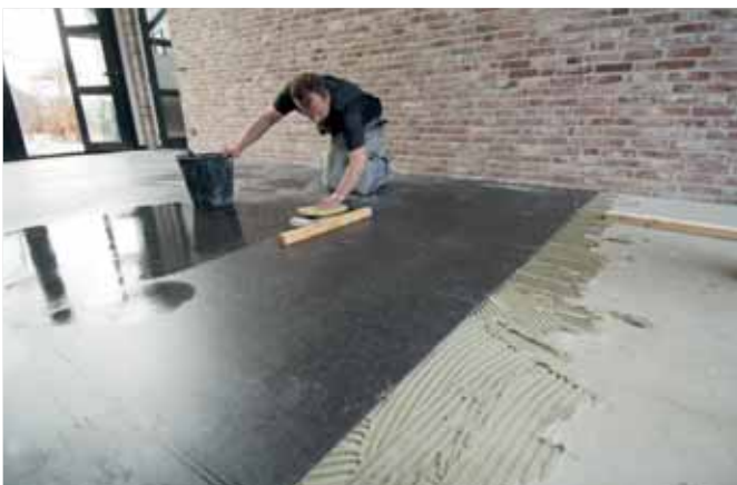
13 Grouting and cleaning 13 Stuccatura fughe e pulizia
