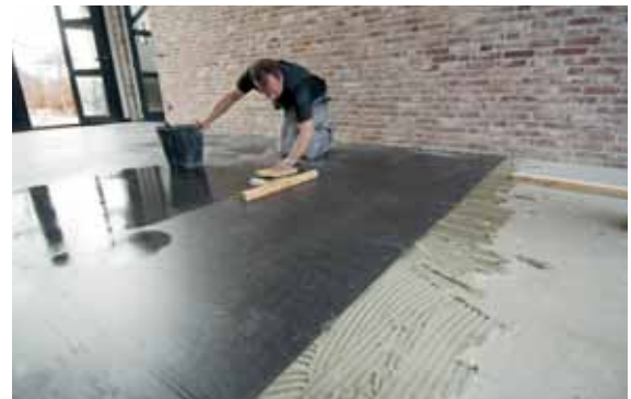
10 Grouting and cleaning 10 Rejuntado y limpieza
